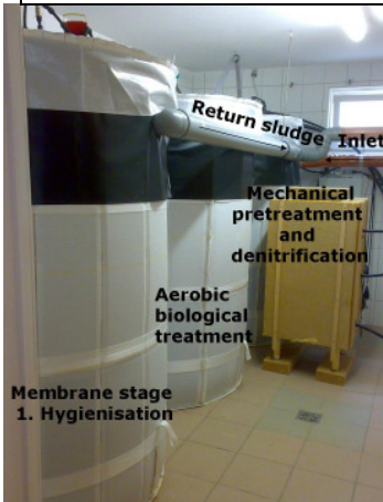
WWTP i. basement 10 p.e. + 3,000 l/d
